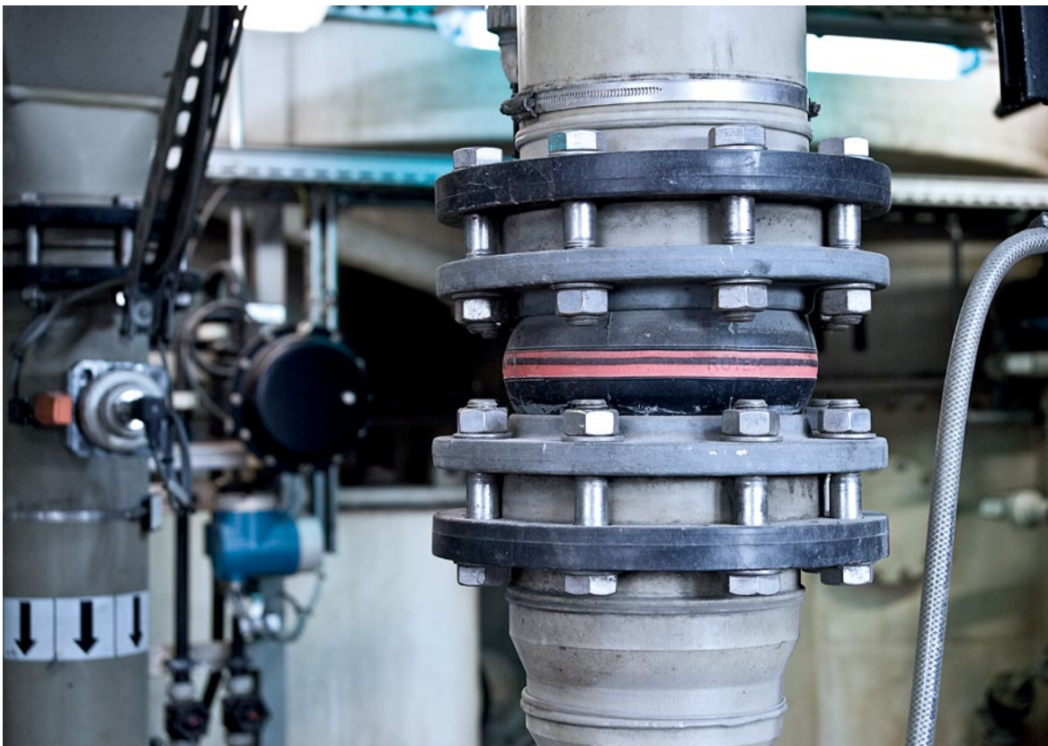
Universal expansion joint, type D110A in a plastic pipe of a paper plant \varnothing 150 mm, design pressure 6 bar
