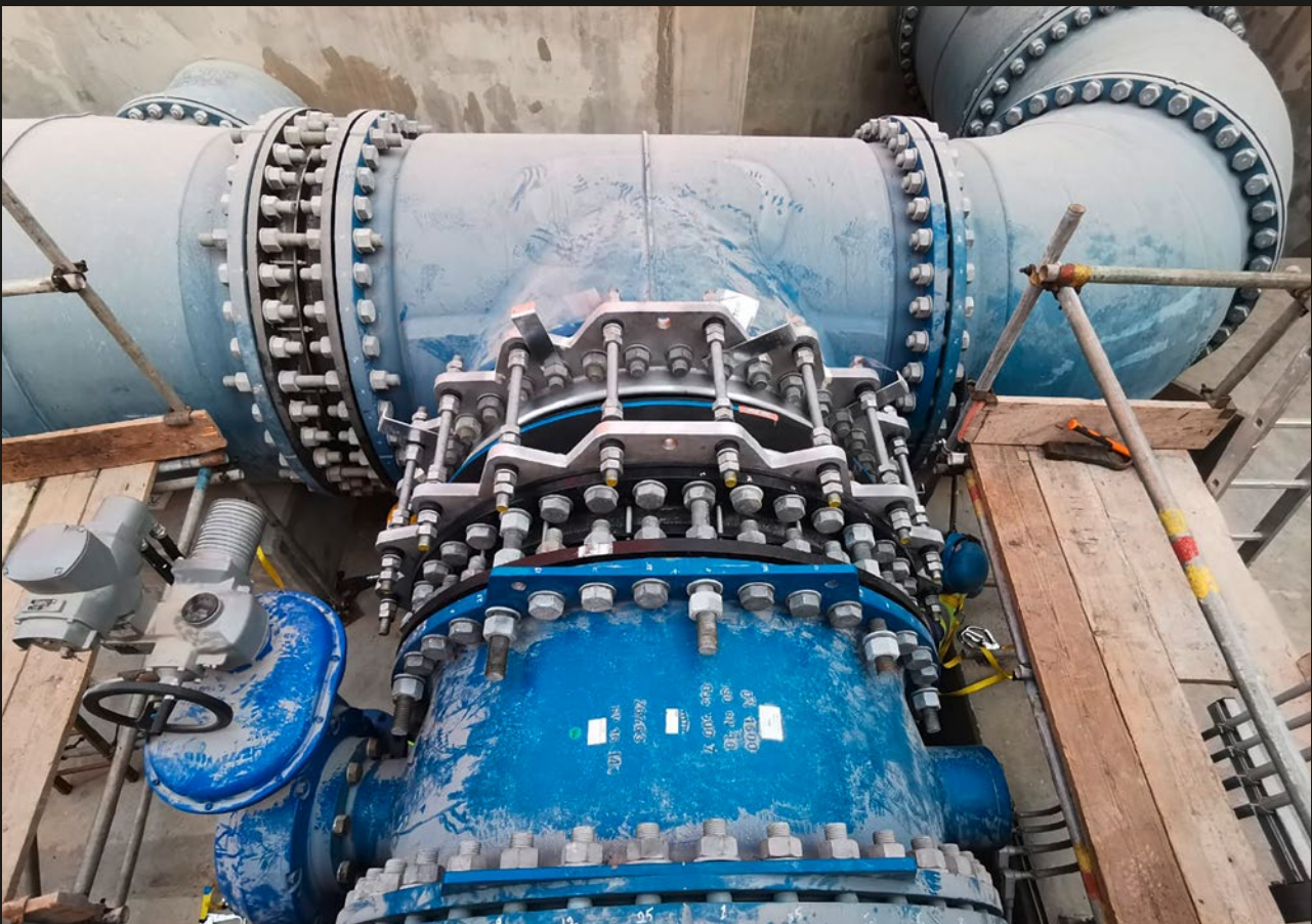
Tied lateral rubber expansion joint with built in angular offset installed in a bypass drinking water line
