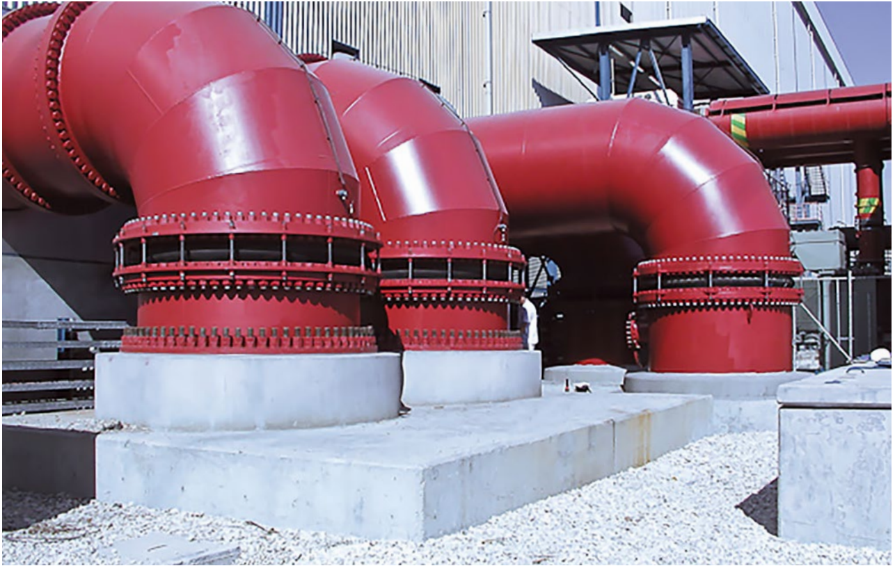
Sea water intake cooling water line \varnothing 2,600 mm, operating pressure 2.5 bar, lateral tied rubber expansion joints of type U111M
