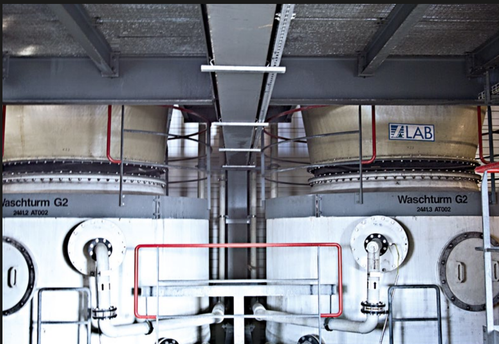
Elastomer expansion joints, type GU100 on the scrubbing drums of a waste incineration plant ∅ 2,400 mm, 80 °C
